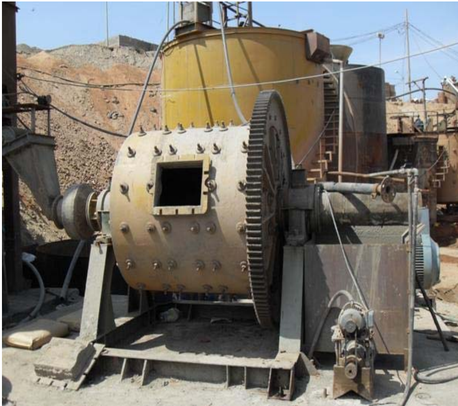
Newly installed ball mill and leaching tanks
