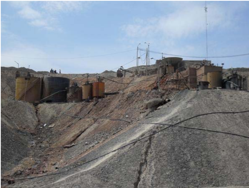
Plant showing new circuit (on the left)
