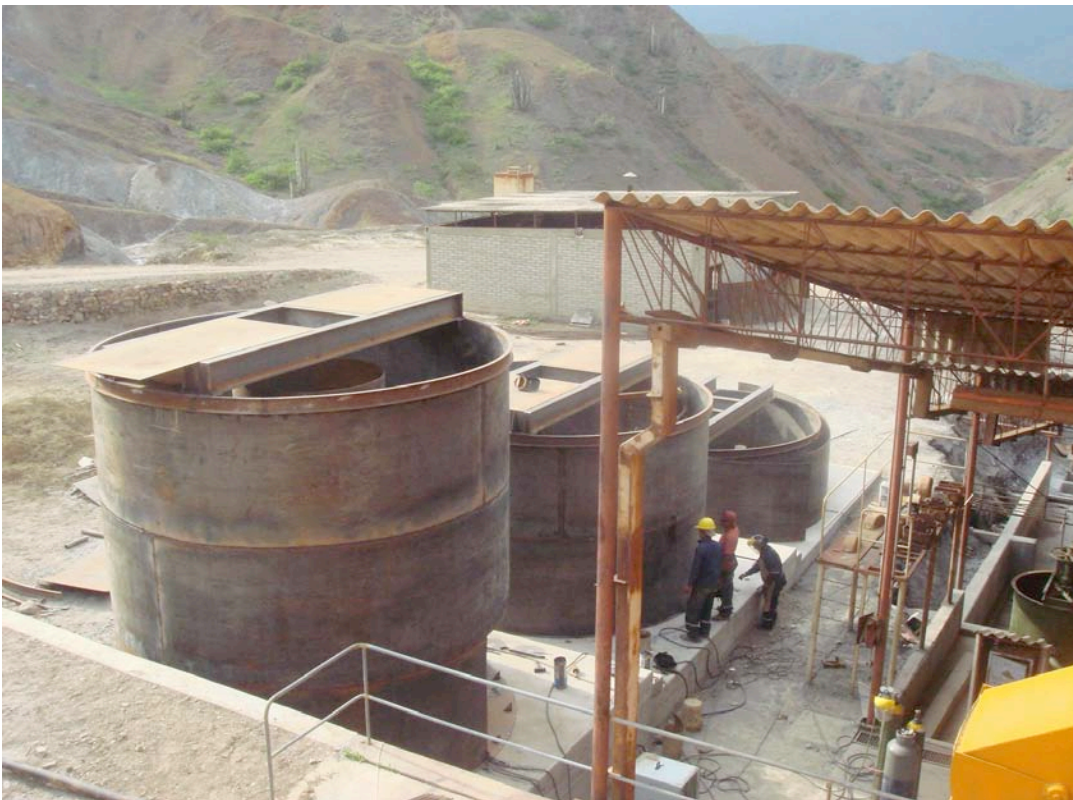
Gold leaching Tanks on their bases at 70% completion
