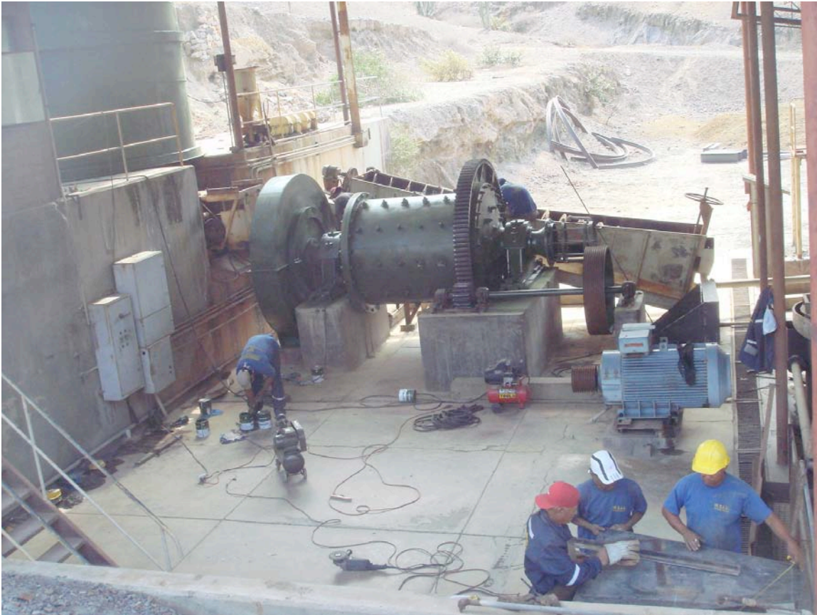
Mechanical work on the ball mill
