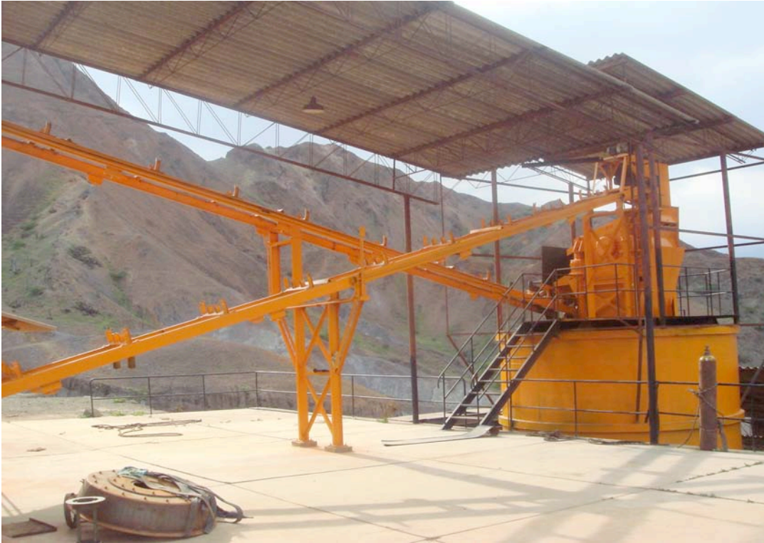
Crushing circuit with fines Bin after overhaul
